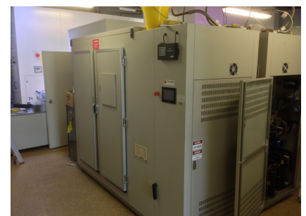
Thermoline Cabinet retrofitted with Andromeda™ Grow Light, Australian National University
