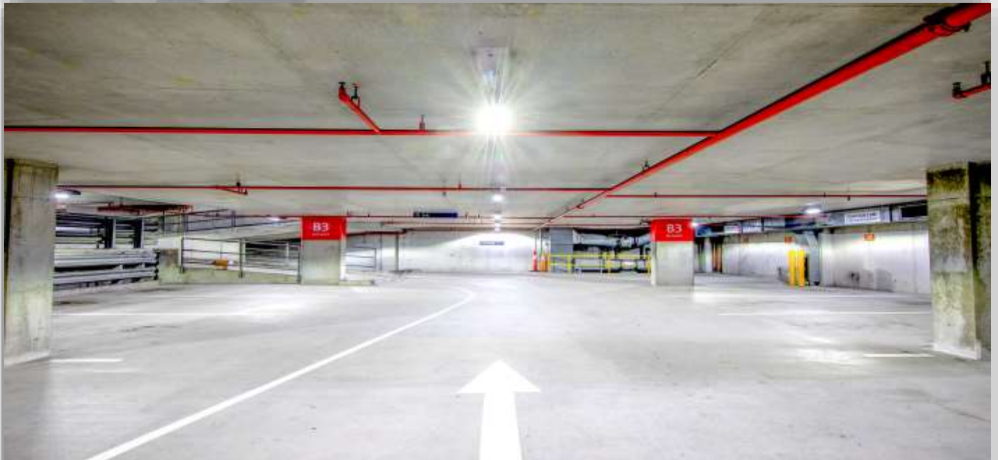
St Andrews War Memorial Hospital – Multi Level Undercover Carpark
